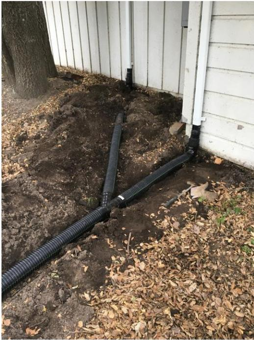
Rain gutter enhancements in Progress
